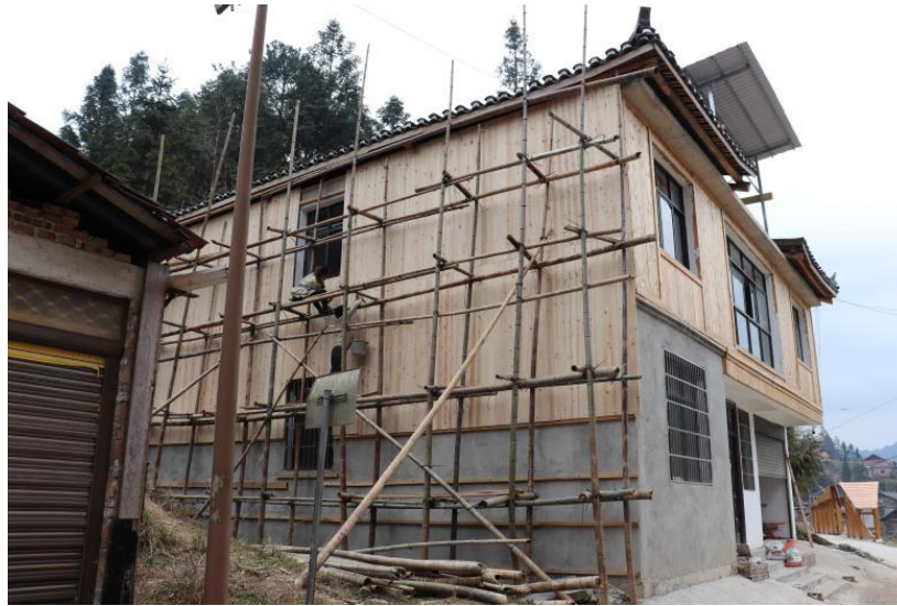
Figure 4. 19 Houses under repair in Zaidang Dong village
