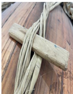
Figure 33 Use wooden pegs to tighten the bamboo gabions
